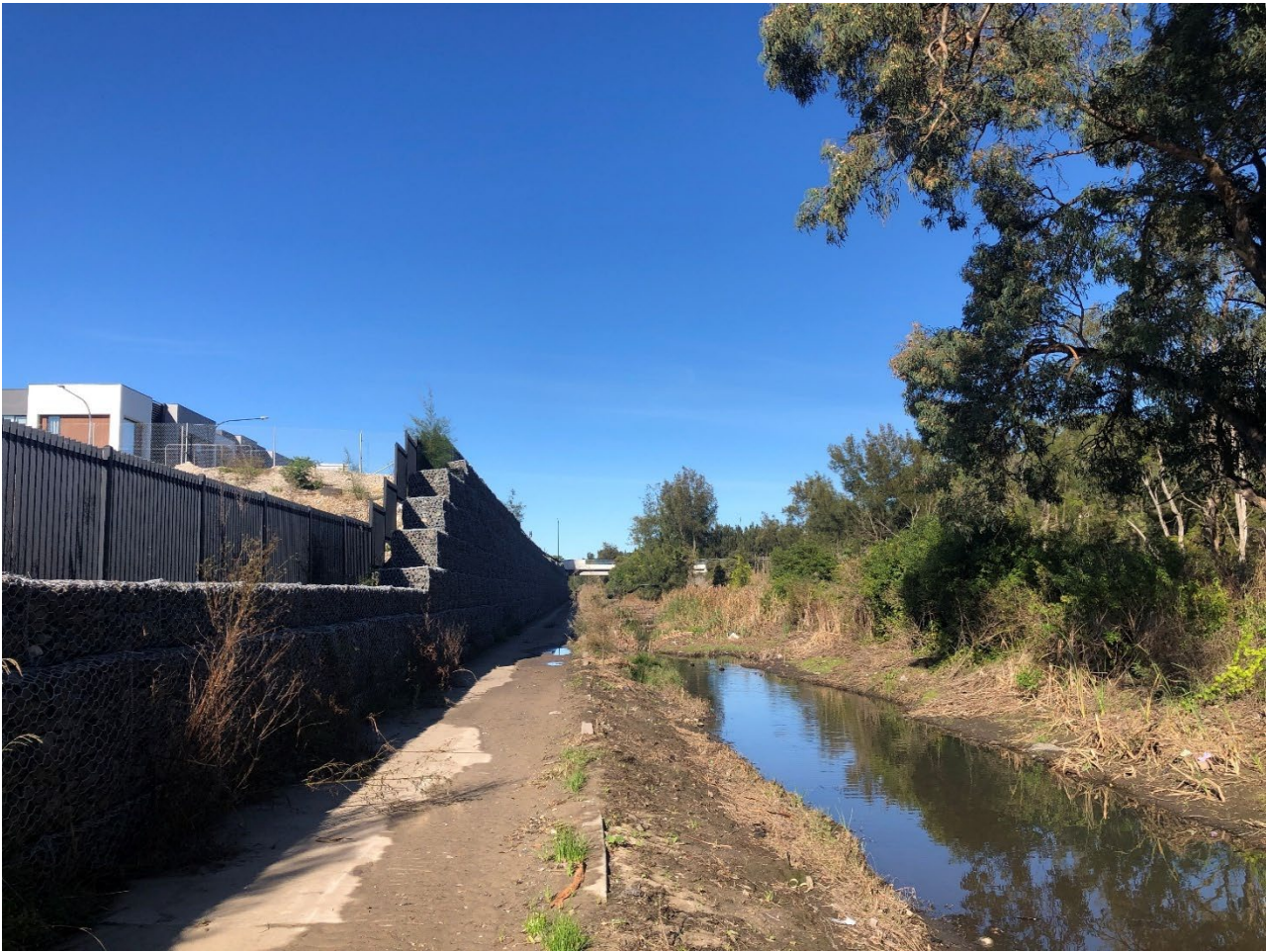
Plate A.4 Further south, looking south along the western boundary of the site, showing the drainage line, the road and the gabion wall.
