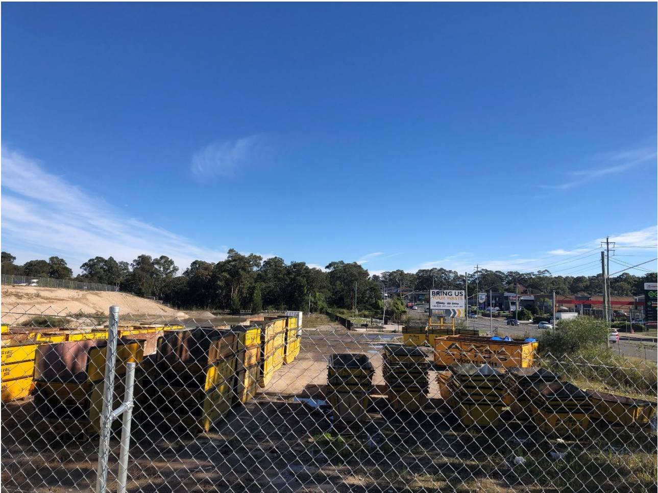
Plate A.7 Looking across the site, standing on the new footpath leading onto Newbridge Road in the north-east corner of the site.
