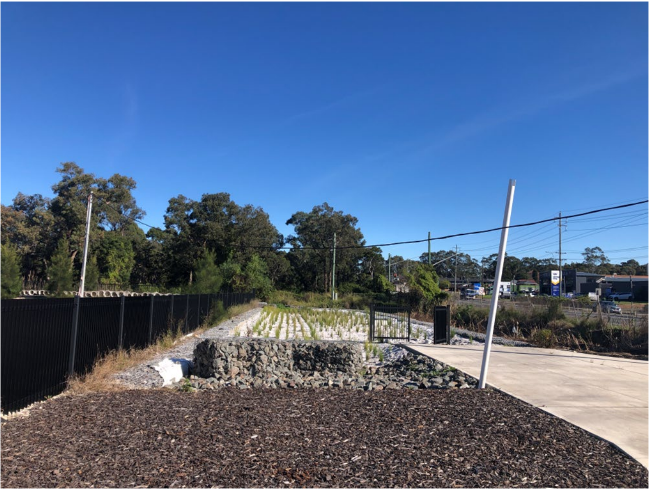
Plate A.1 Looking west, at the new raingarden, and drainage channel area (to the north of the Rain Garden) between Newbridge Road and the Rain garden
